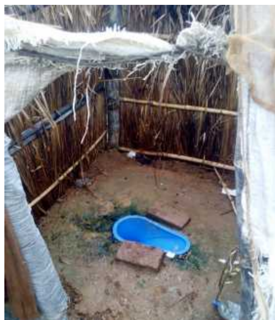
A household latrine in Rangamati built with SATO pan; Photo: Enamul Kabir
