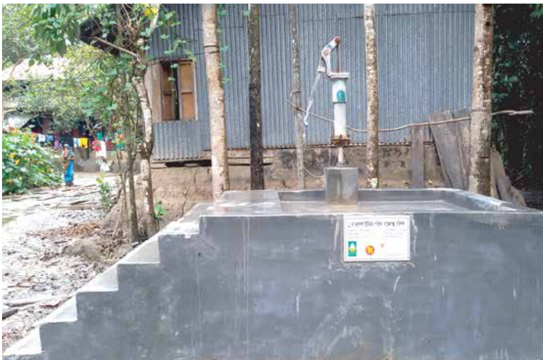
HYSAWA has installed tube-wells on raised platform in order to build resilience to climate change
