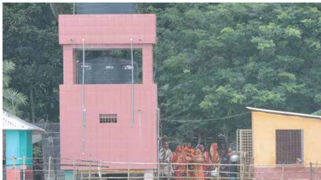
Sky hydrant, a water purification system, provides people with safe drinking water in geo-physically difficult areas
