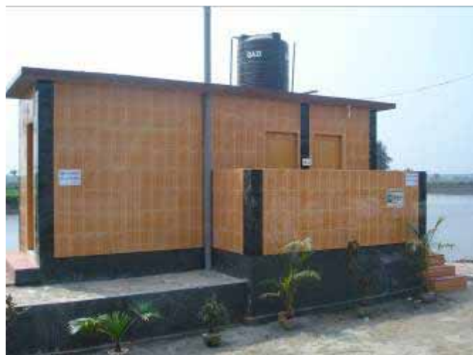
A three chamber institutional latrine installed at Khulna
