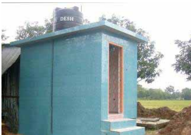
A two chamber institutional latrine installed at Naogaon
