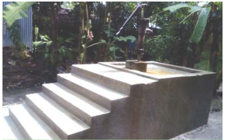
A raised-platform tube well constructed by HYSAWA under climate change adaptation programme.
