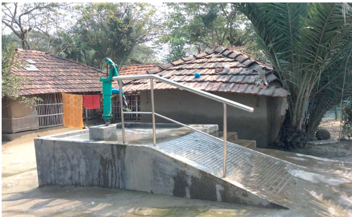
HYSAWA has installed tubewells on raised platform in order to build resilience to climate change and make it disable friendly
